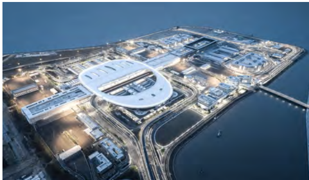
Hong Kong-Zhuhai-Macao Bridge
